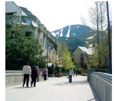
pedestrian bridge south
