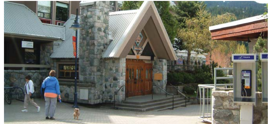
south-west view (Restrooms and Restaurant)
